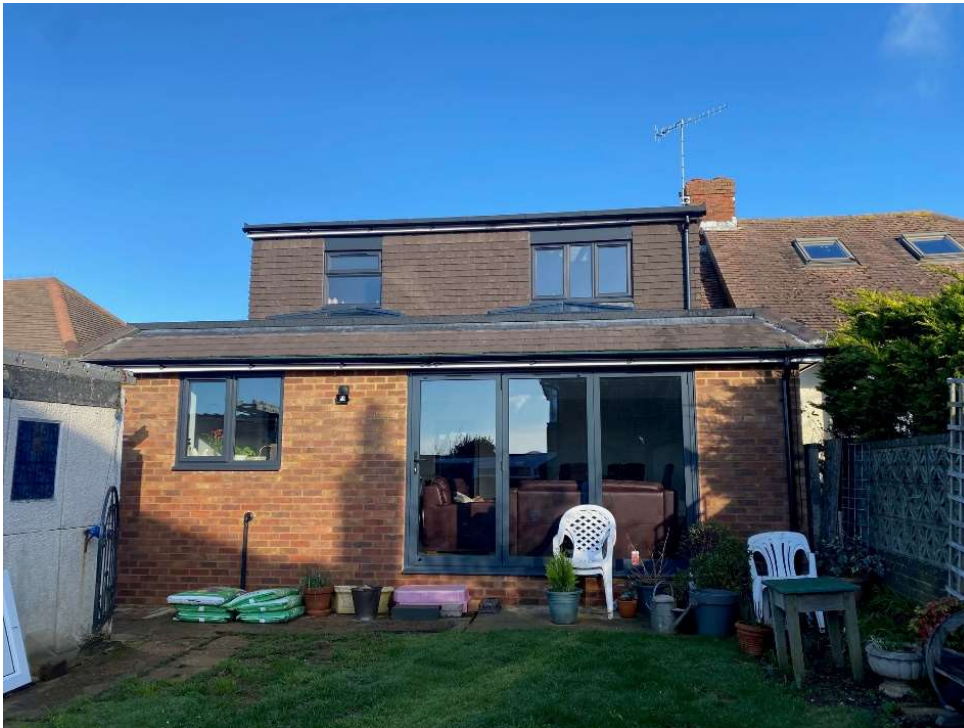
Rear (southern) elevation of no. 14 (site)
