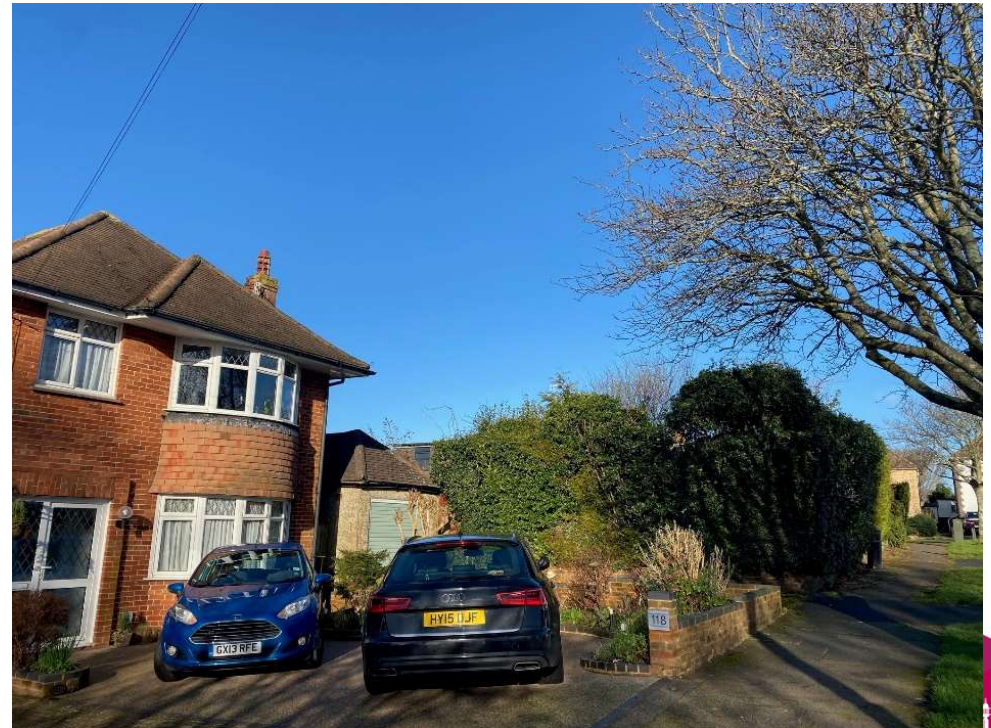
View of dormer from Foredown Drive
